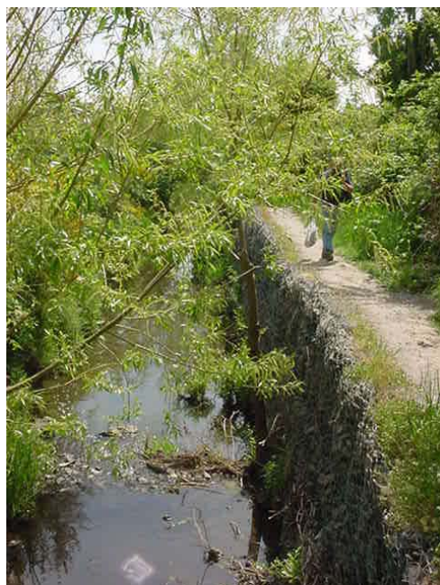
Figure 5: West Bank—Gabion Wall
